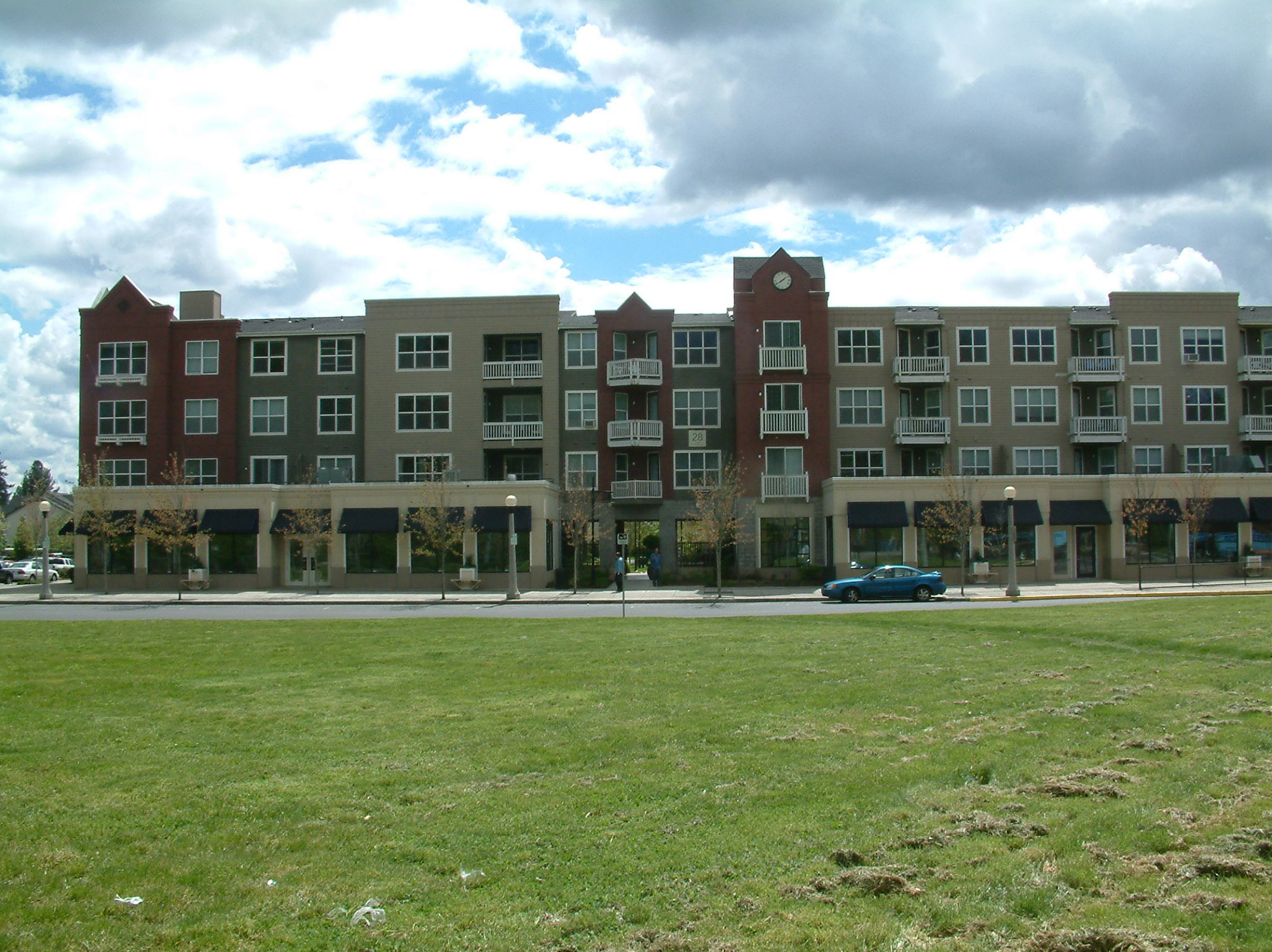
Here is a mixed-use development with apartments on the top three stories and space for shops on the ground floor. But every single shop you see in this photo
