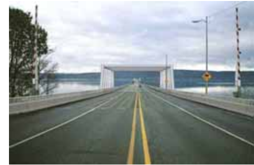
$45.8M/Mile SR 104 Hood Canal Bridge East-half Replacement and West-half Retrofit Project, Washington
