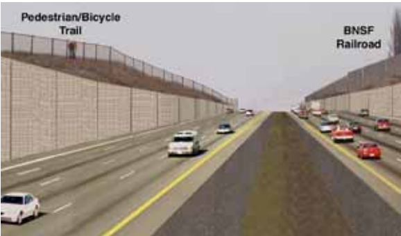
$9M/Mile US 395 North Spokane Freeway - Spokane, WA
