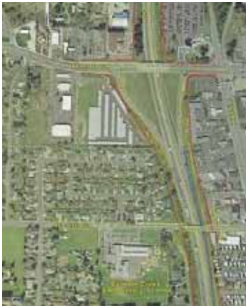
$9.3M/Mile I-5 Widening Salmon Creek to 205 - Vancouver, WA
