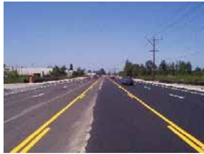
$3.8M/Mile SR 525 Widening & Safety - Mukilteo, WA
