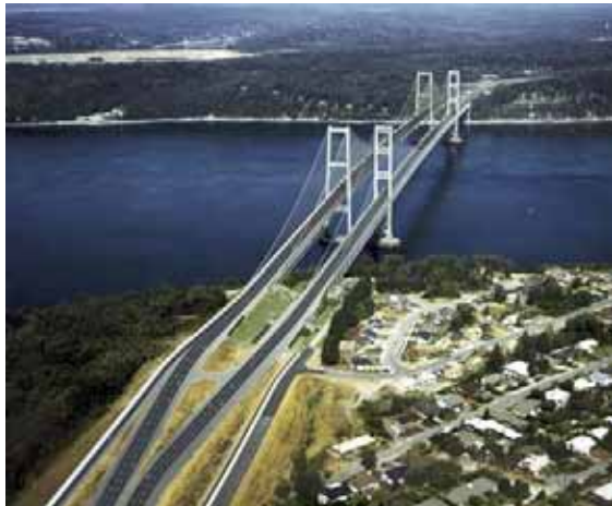
$67.2M/Mile Tacoma Narrows Bridge – Tacoma, Washington
