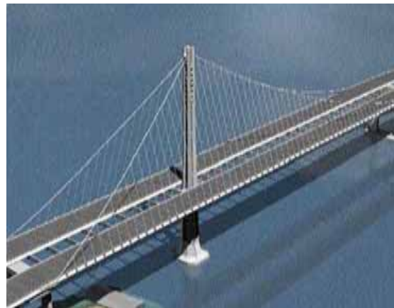
$64.2-$82.6 M/Mile Oakland Bay Bridge - San Francisco, California
