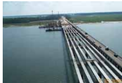
$4.4M/Mile SC 170 Widening - Beaufort, SC
