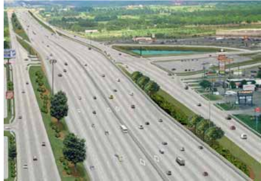
Katy Freeway at Fry Road after
