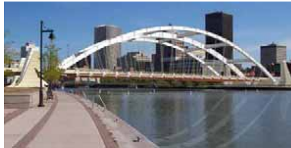
$27.8M/Mile Troup Howell Bridge - Rochester, New York
