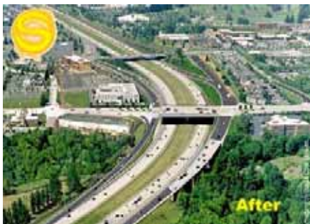
$28M The Sunnybrook Boulevard Interchange - Clackamas County, Oregon
