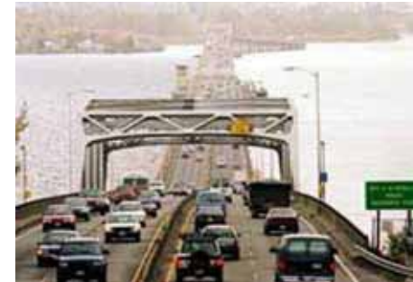
$45.6-$52.9M/Mile SR 520 Bridge Replacement & HOV - Seattle, WA
