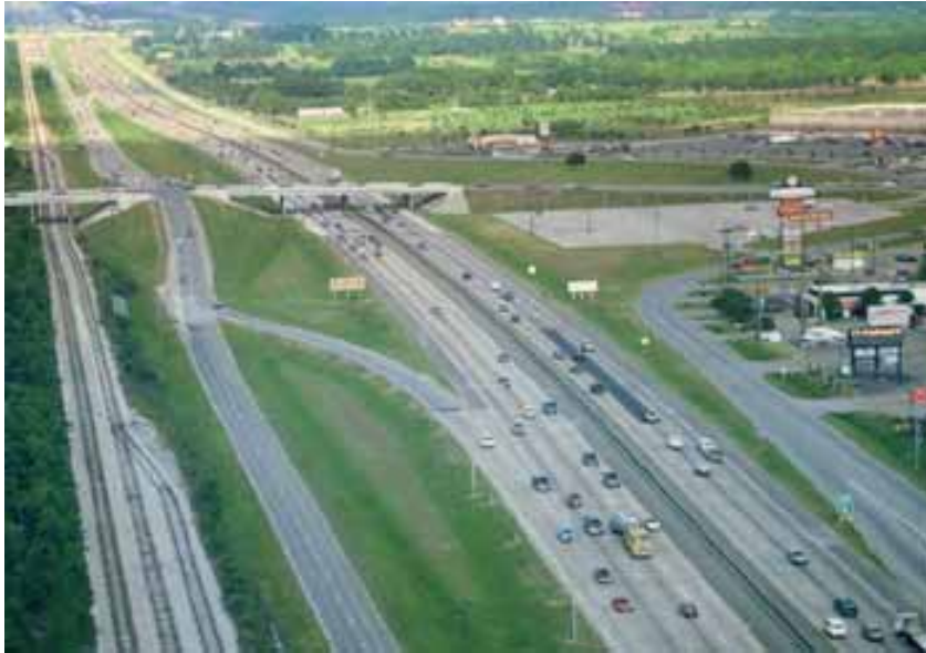
Katy Freeway at Fry Road before
