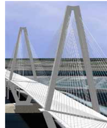
$278M/Mile Cooper River Bridge Project - Charleston, South Carolina
