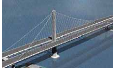
$64.2-$82.6M/Mile Oakland Bay Bridge - Oakland, CA
