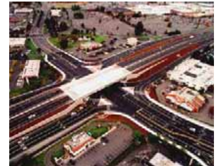
$26.8M SR 500, Thurston Way Interchange - Vancouver, Washington
