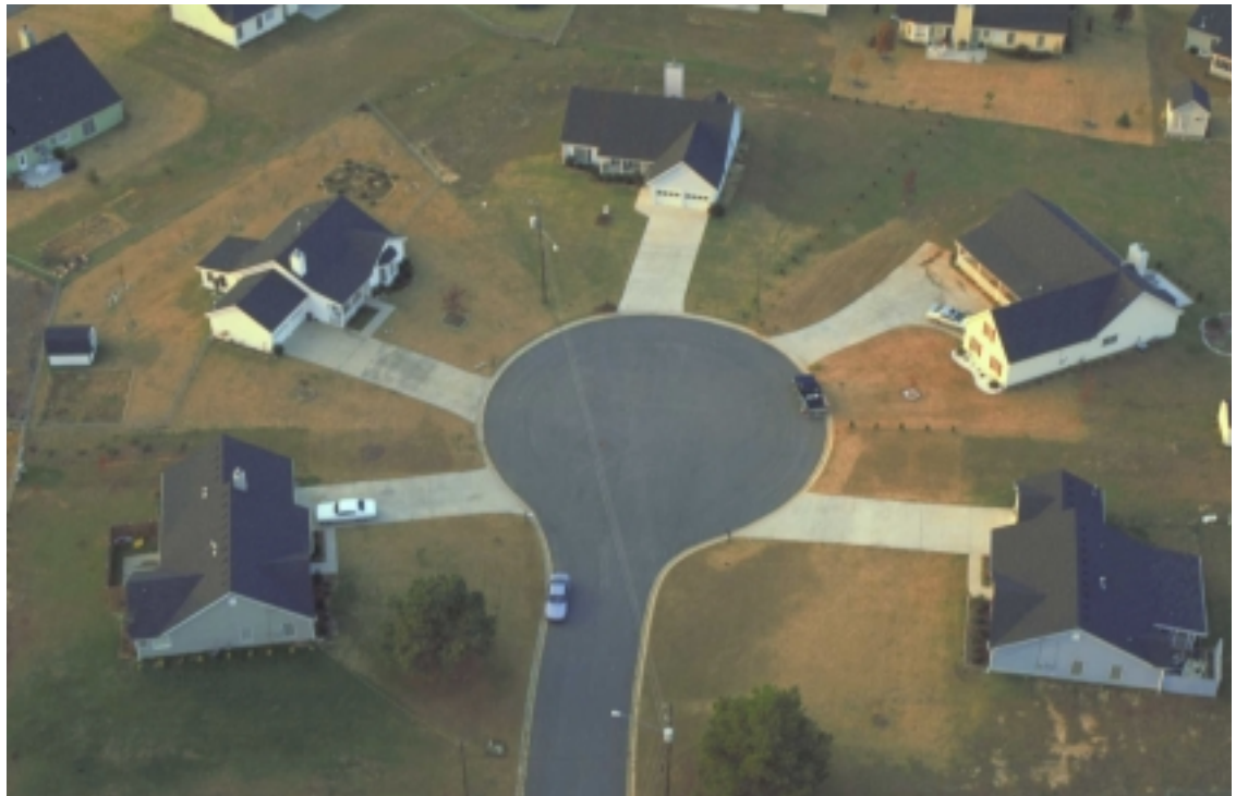
Figure 11: A Suburban Subdivision
