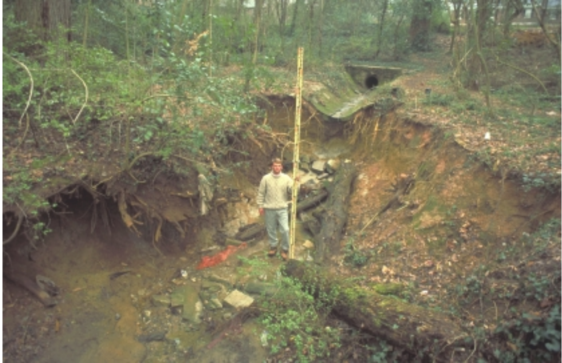
Figure 4: Stormwater Culvert Carrying Road Runoff Into the Head of the Stream Draining the Deepdene Watershed
