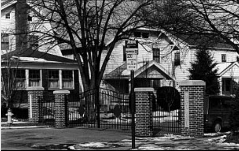
Figure II-18: Gates as actually installed.
