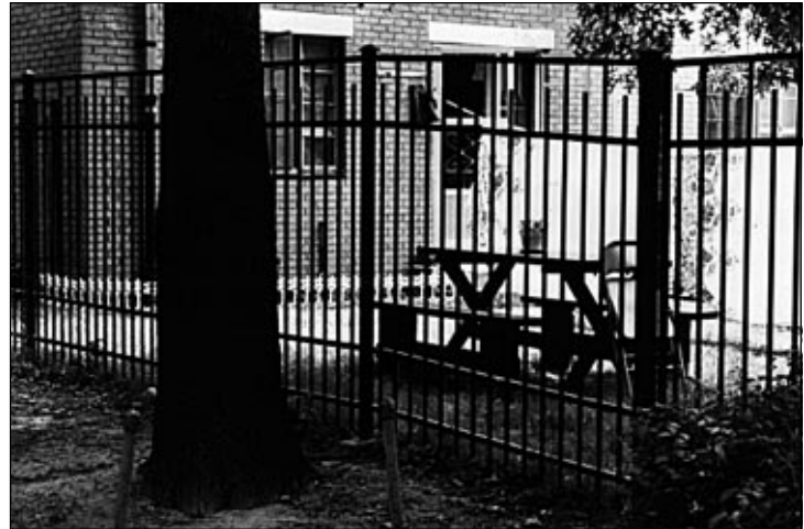
Figure III-4: Six-foot-high tubular steel fencing defines the collective rear yards of residents, allowing them to place picnic tables and other outdoor furnishings there for the first time.
