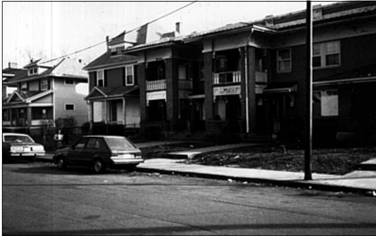
Figure II-3: Deteriorated two-story walkup in Five Oaks being rented to drug dealers.
