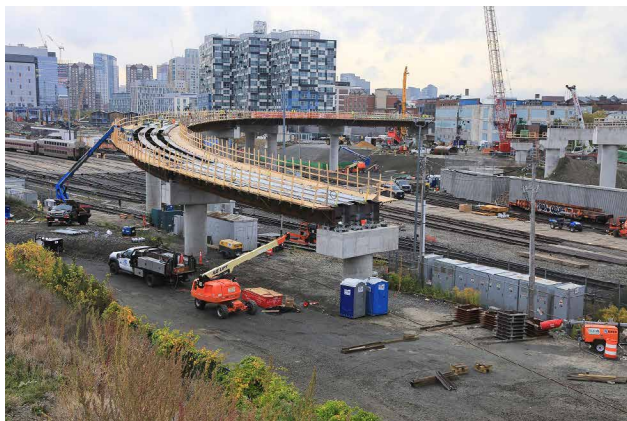
The Green Line Extension under construction. Though entirely above ground, this light-rail line is costing $500 million per mile. Photo from Massachusetts Department of Transportation.
