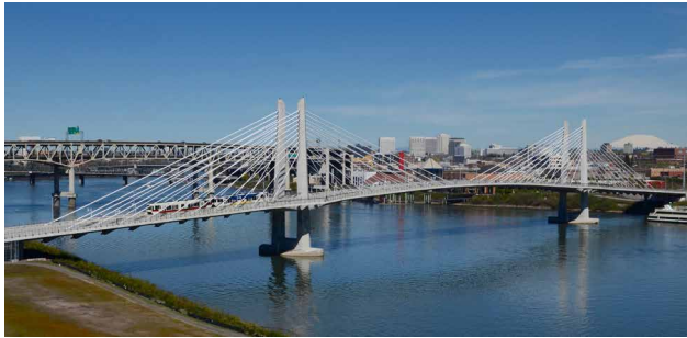
A new bridge added $135 million to the cost of the Orange Line, but this was only about 10 percent of the difference in costs between it and the original Blue Line. Photo by Steve Morgan.
