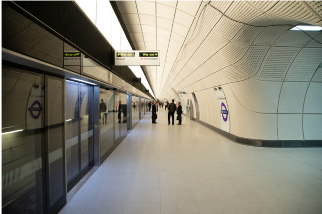
Platform screens at Farringdon Station on London's Crossrail line. Photo by Tom Page.
