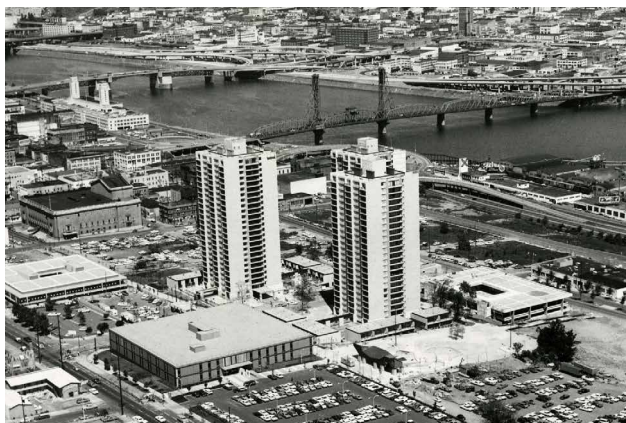
These are the first three of six luxury high rises built to replace a low-income neighborhood south of downtown Portland. Portland claims this is only the second use of TIF for any project in the United States.
