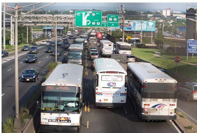
The line of buses on the left are headed for the Lincoln Exclusive Bus Lane, which moves as many as 25,000 people per hour. Photo from the state of New Jersey.
