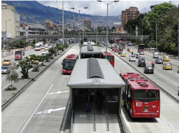
Bogotá's Transmilenio is estimated to have the highest capacity of any bus-rapid transit line in the world, partly because there are passing lanes for express buses. Photo by EMBARQ.
