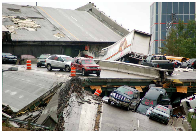
Minnesota's I-35 bridge collapse in 2007 led many to call for more infrastructure spending. But the NTSB report about the failure found that it was due to a design flaw that could not have been detected by routine inspections and maintenance. Coast Guard photo by Kevin Rofidal.
