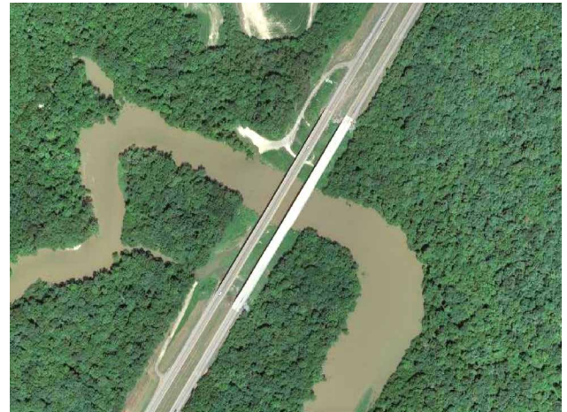
The Hatchie River Bridge, the last U.S. road bridge to fail due to inadequate maintenance. The light pavement shows the part that collapsed in 1989 and was replaced.
