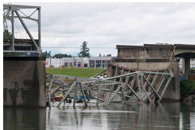
The failure of the I-5 bridge across Washington's Skagit River led to more calls for infrastructure spending. But the NTSB report about the collapse found that it was solely due to an oversized vehicle that should not have attempted to cross the bridge; the bridge would have failed if that vehicle had attempted to cross on the day it opened. Photo by kdingo.
