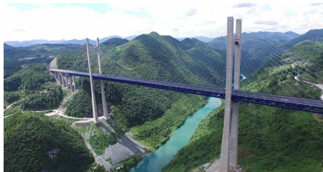
The Gongsuihe Bridge deck is 850 feet above the river and the span between the two towers is 1,300 feet long. Photo by HighestBridges.com.
