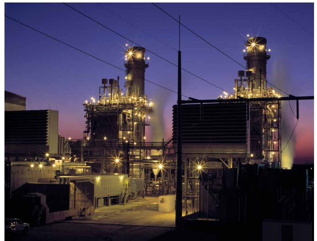
A natural gas power plant in South Carolina. Photo courtesy of the American Public Power Association.
