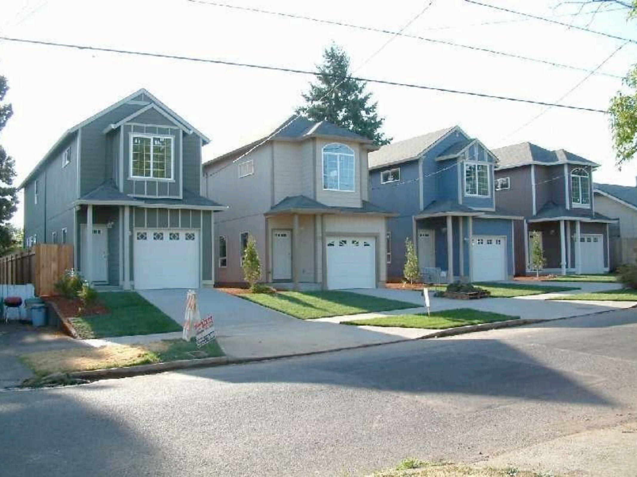
And replace them with four “skinny houses,” houses just 15 feet wide on 25-foot-wide lots.
