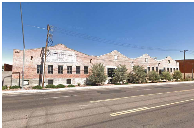
KSport, an auto parts company, is located in this building a mile away from a light-rail line, yet Valley Metro claims it was stimulated by light rail.
