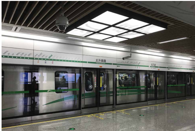
The Chengdu Metro has clear walls and doors that protect passengers from suicide or accidentally falling onto tracks. Photo by Asuracd.
