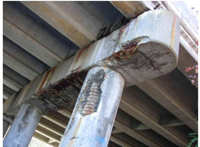
The number of bridges in poor condition declined from nearly 138,000 in 1990 to under 44,000 in 2021. Photo by Richard Klein.
