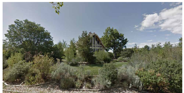
The trees and vegetation around this home, located not far from the one in the previous photo, were enough to ensure its destruction.
