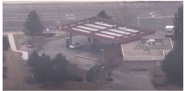
This gasoline station survived while nearby homes did not, demonstrating the value of firewise design.
