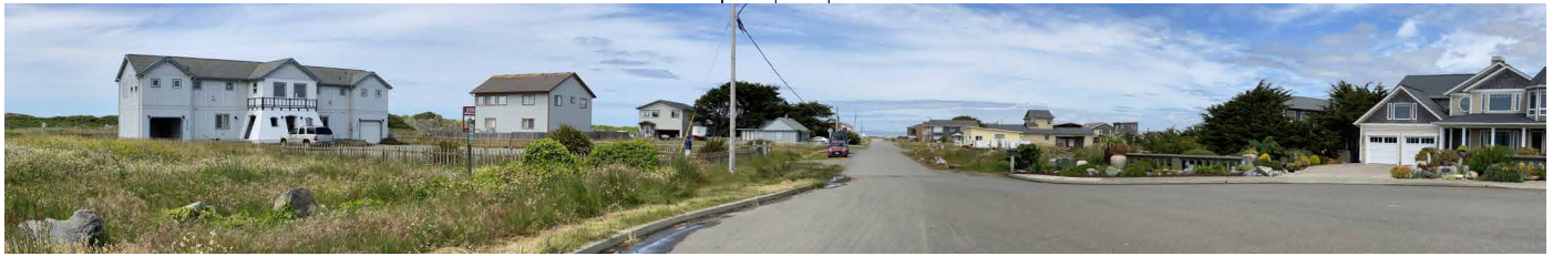
This Bandon neighborhood includes about two dozen homes, ten of which front on the ocean. None would have been allowed by the Freeman plan.
