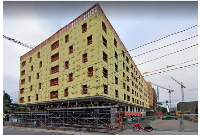
The Broadway TOD, now under construction in Seattle.
