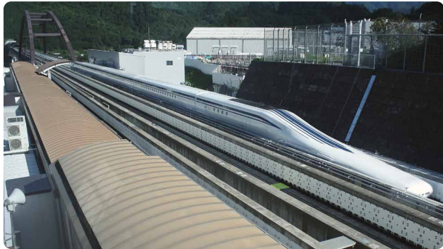
Construction has begun on some of the tunnels for a maglev line that will cost five times as much money and use five times as much energy to operate as the parallel Tōkaidō Shinkansen. Photo by Saruno Hirobano.
