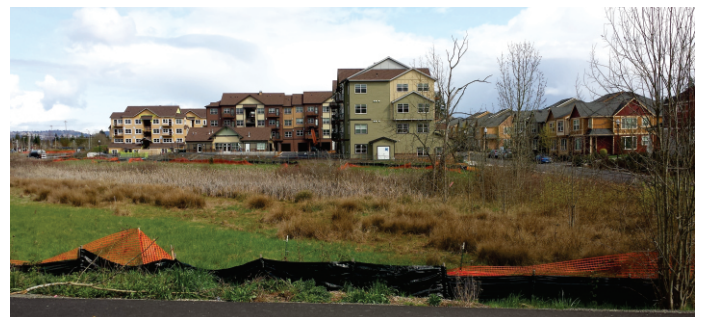
This open space near Elmonica light rail station must be filled in with high-density housing to comply with zoning requirements.
