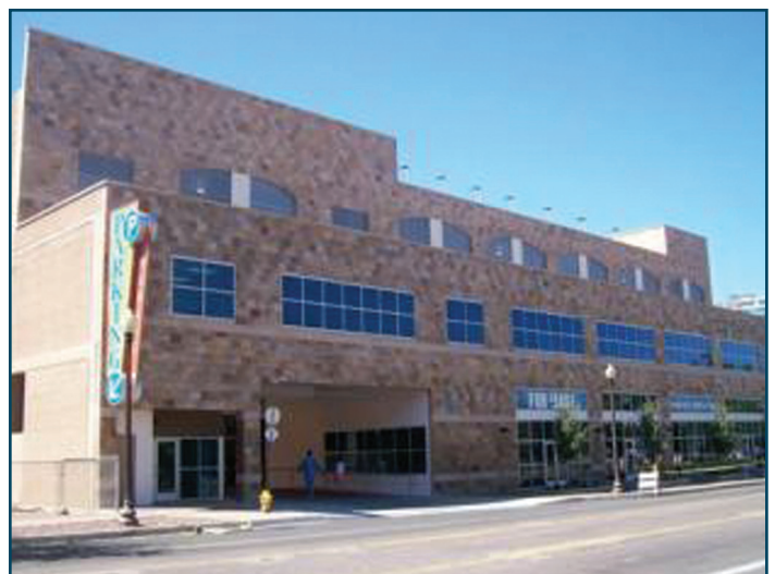
Tempe City Hall Parking Garage
