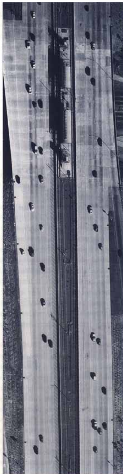
Century Freeway with Green Line and station in the median.
