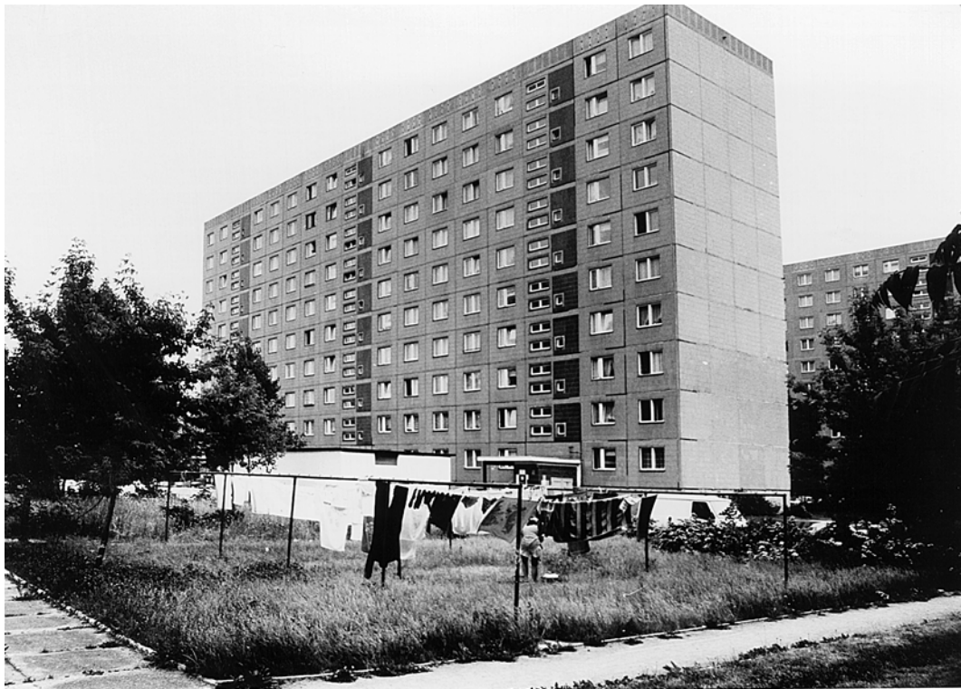
Fig. 4 Unshaped area between individual (Apartments in residential block, QP 71) and societal (area for laundry drying) space in Berlin-Marzahn
