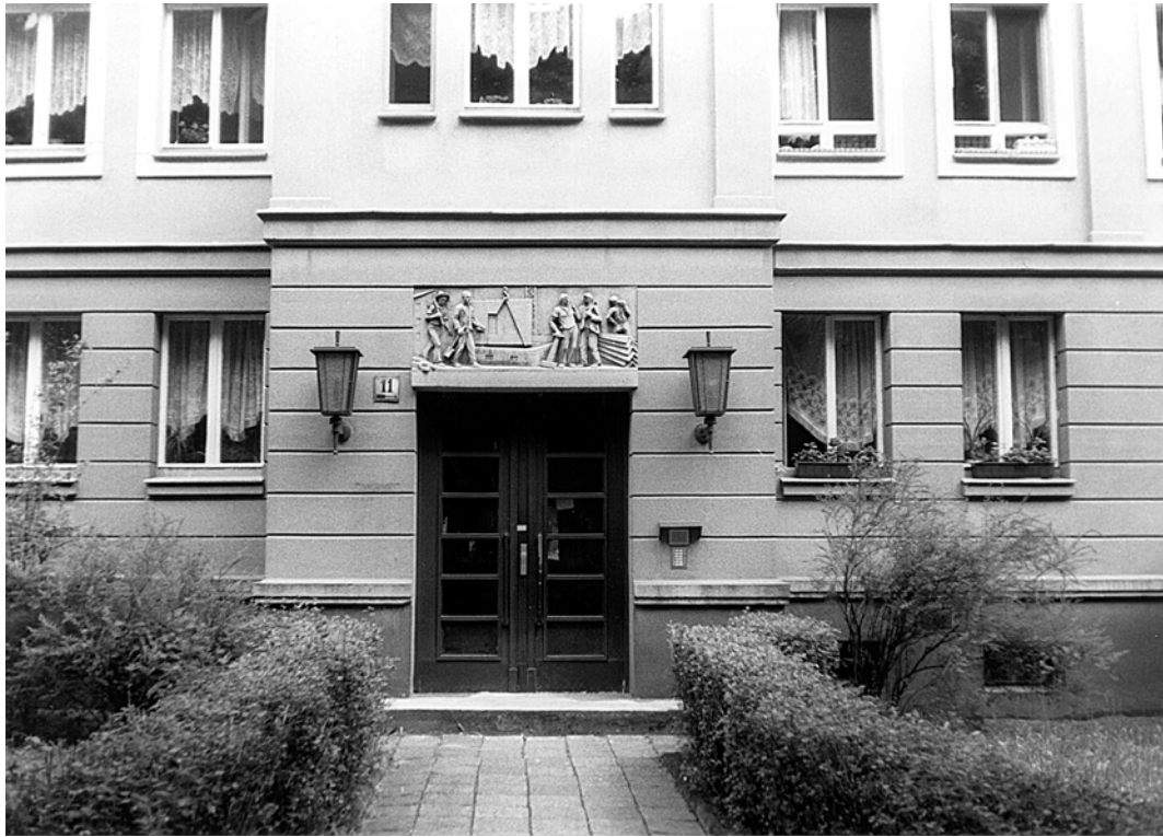
Experimental building in large panel construction of 1953 in Berlin-Johannisthal (above: entry; below: backside)
